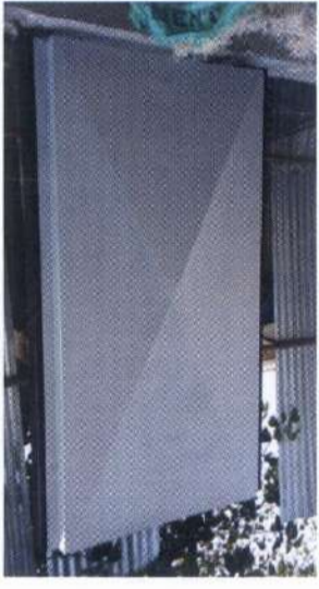
Opposite page: view of the staircases, and the entrance to the design studio. This page, left: detail of the compound wall. Below: 0.6mm-thick Galvalume sheet being used for the compound wall. The material can easily withstand being exposed to direct rain, adding to longevity
